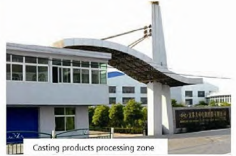
Casting products processing zone
