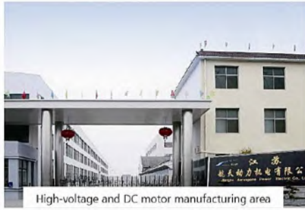
High-voltage and DC motor manufacturing area
